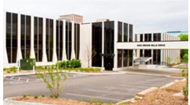
South Side of Building
